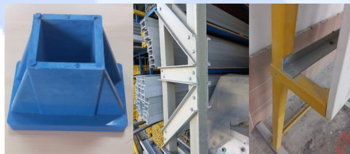
Figure 4. Connection details of GFRP profiles
