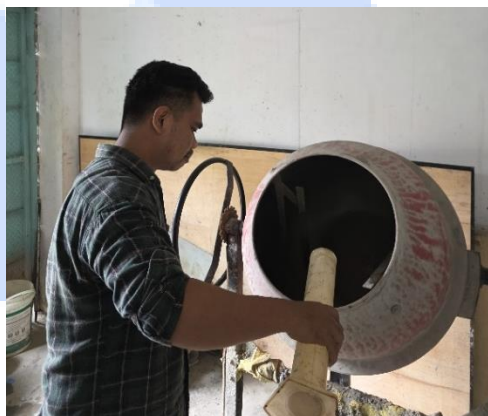
Figure 1. Mixing of SCC materials using a concrete mixer
